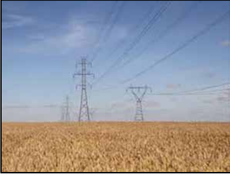
The AltaLink transmission lines are situated at the north end of the reserve.
