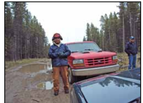
The workers, many from Moses Lake, cut rails despite the wet weather conditions.
