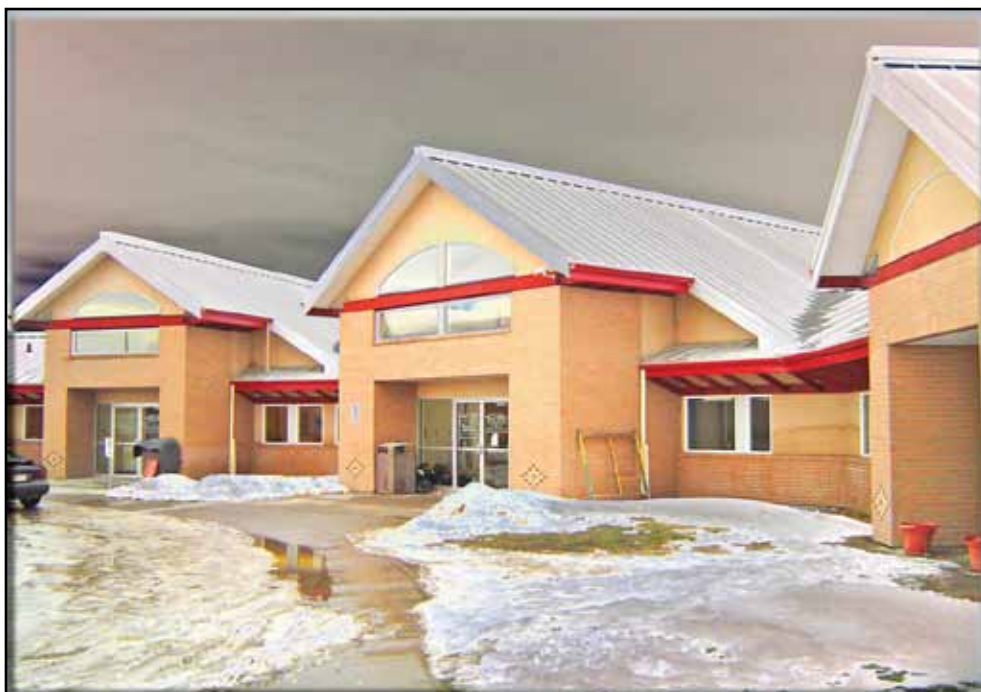
The Family & Community Support Services is housed in the Human Resources facility.
