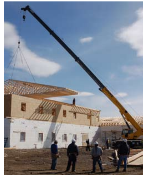
Construction of multi-purpose building in Lavern. Raising the roof. Aug.06
