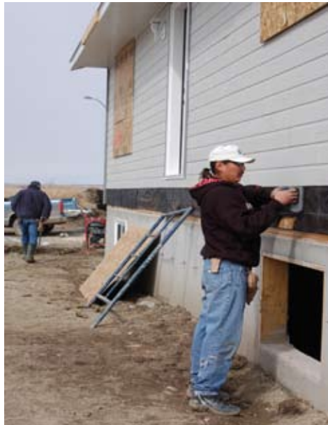
Construction on new home in Lavern Community, much needed housing.
