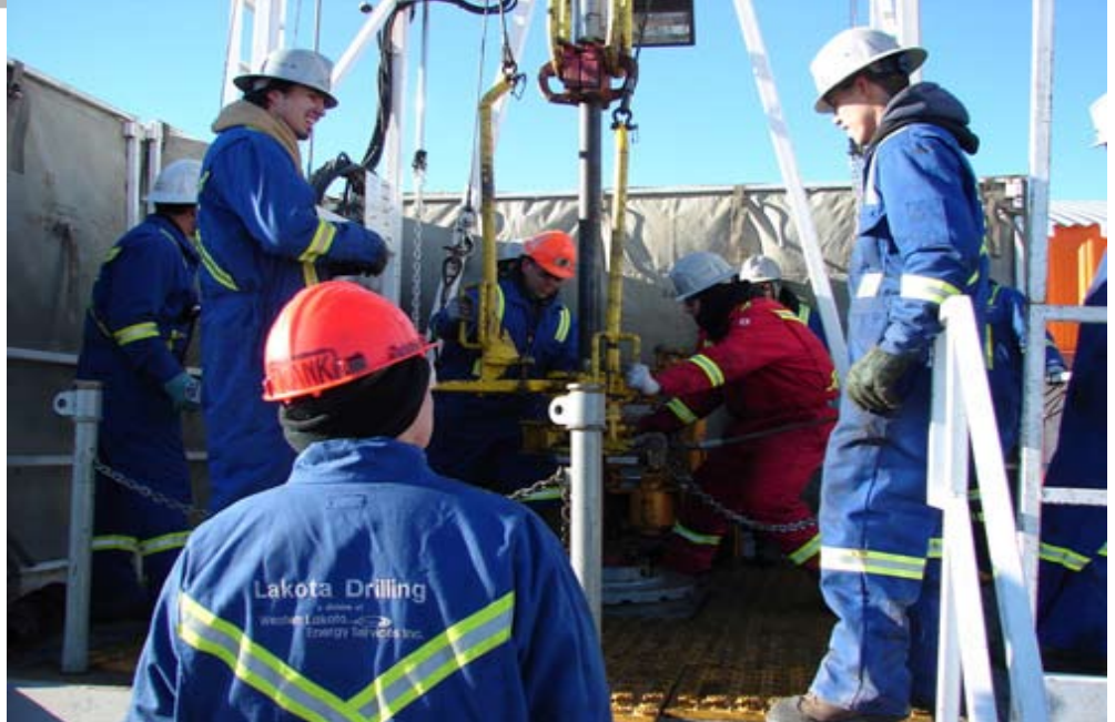
Graduates from the Aboriginal Drilling Rig Training Program during drilling demonstration
